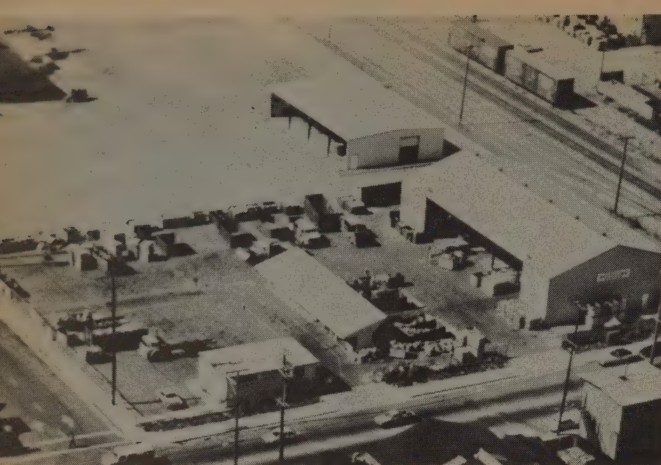
▲ Berkeley's Solid Waste Transfer Station before it opened in 1982. The empty area in the background was to have housed the burner which was never built. Instead it became the site of the Flea Market.
